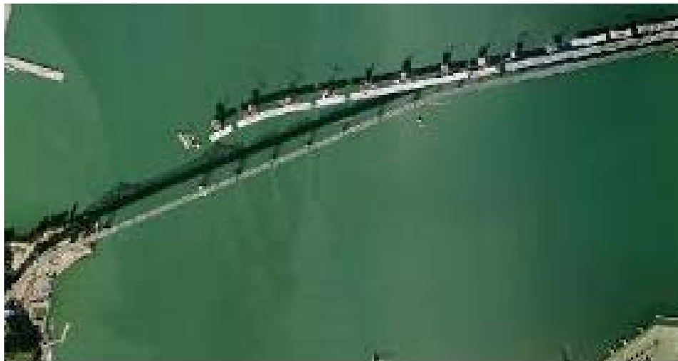
Figure 2. Aerial photo of construction area (Terra Server 2007)
